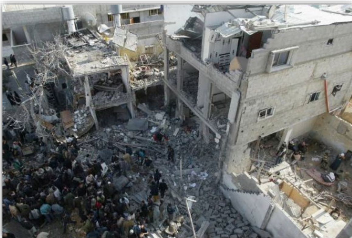
Figure 6 Destruction of homes in al-Bureji on 3 March 2003 Photo: © Fayez Nureldine/AFP via Getty Images
